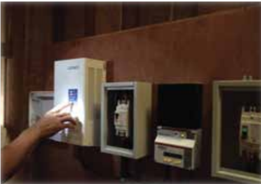
Solar Home Systems
